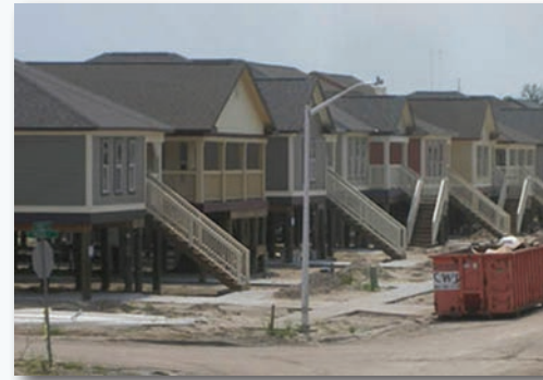
Construction of homes in Jefferson Parish, LA. Credit: Louisiana Recovery Authority
